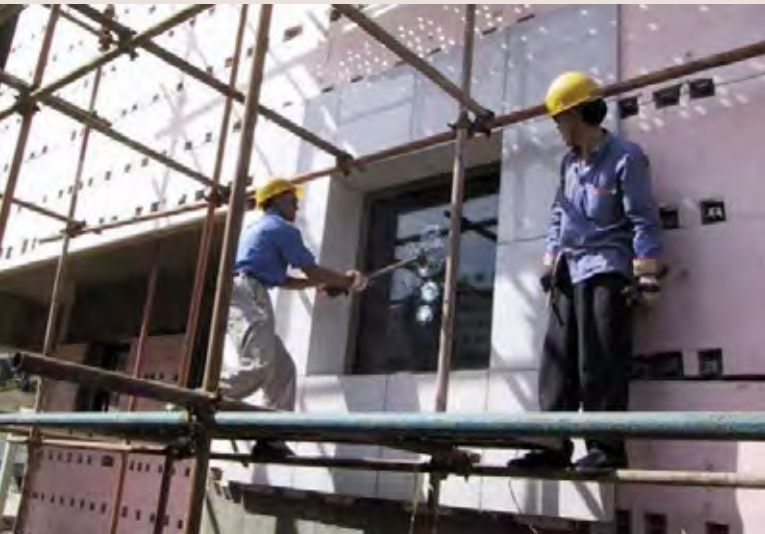
Figure 38: Testing of 15 minutes forced entry resistant window
