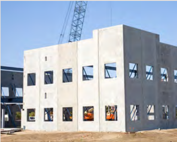
Figure 23: Building constructed from pre-cast elements
