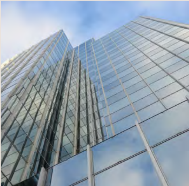
Figure 24: Example of fully framed curtain wall
