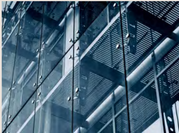
Figure 25: Example of a point supported curtain wall
