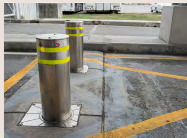
Figure 14: Retractable anti-ramming bollards
