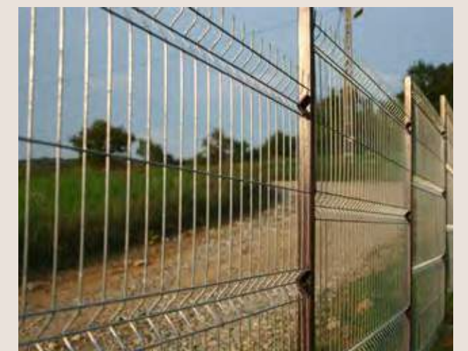
Figure 10: A welded mesh fence
