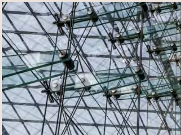
Figure 26: Example of a point support
