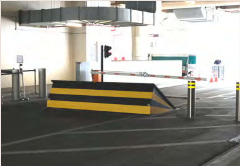
Figure 2: A crash-rated wedge vehicle security barrier.
