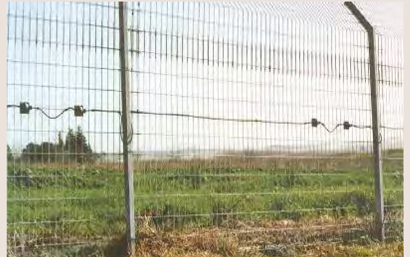
Figure 9: A welded mesh fence with sensor line
