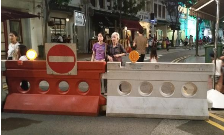
Figure 6 Example of how blinker is installed
